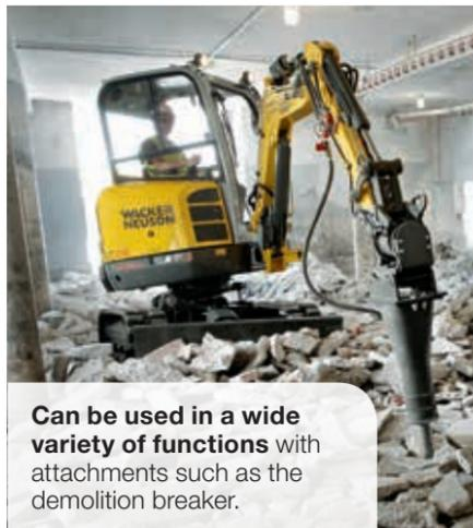
**Can be used in a wide variety of functions** with attachments such as the demolition breaker.
