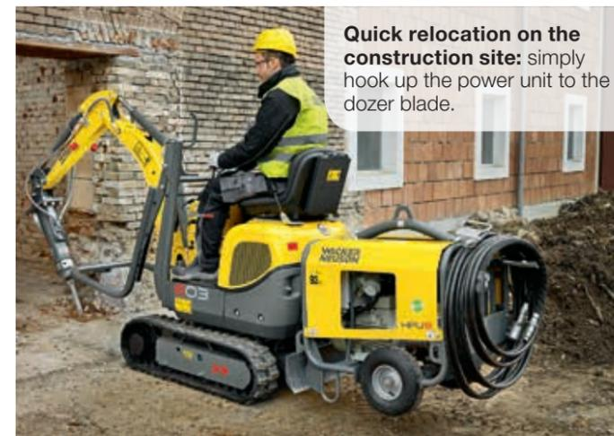
**Full freedom of movement, zero emissions:** flexible set-up options for interior demolition work.
